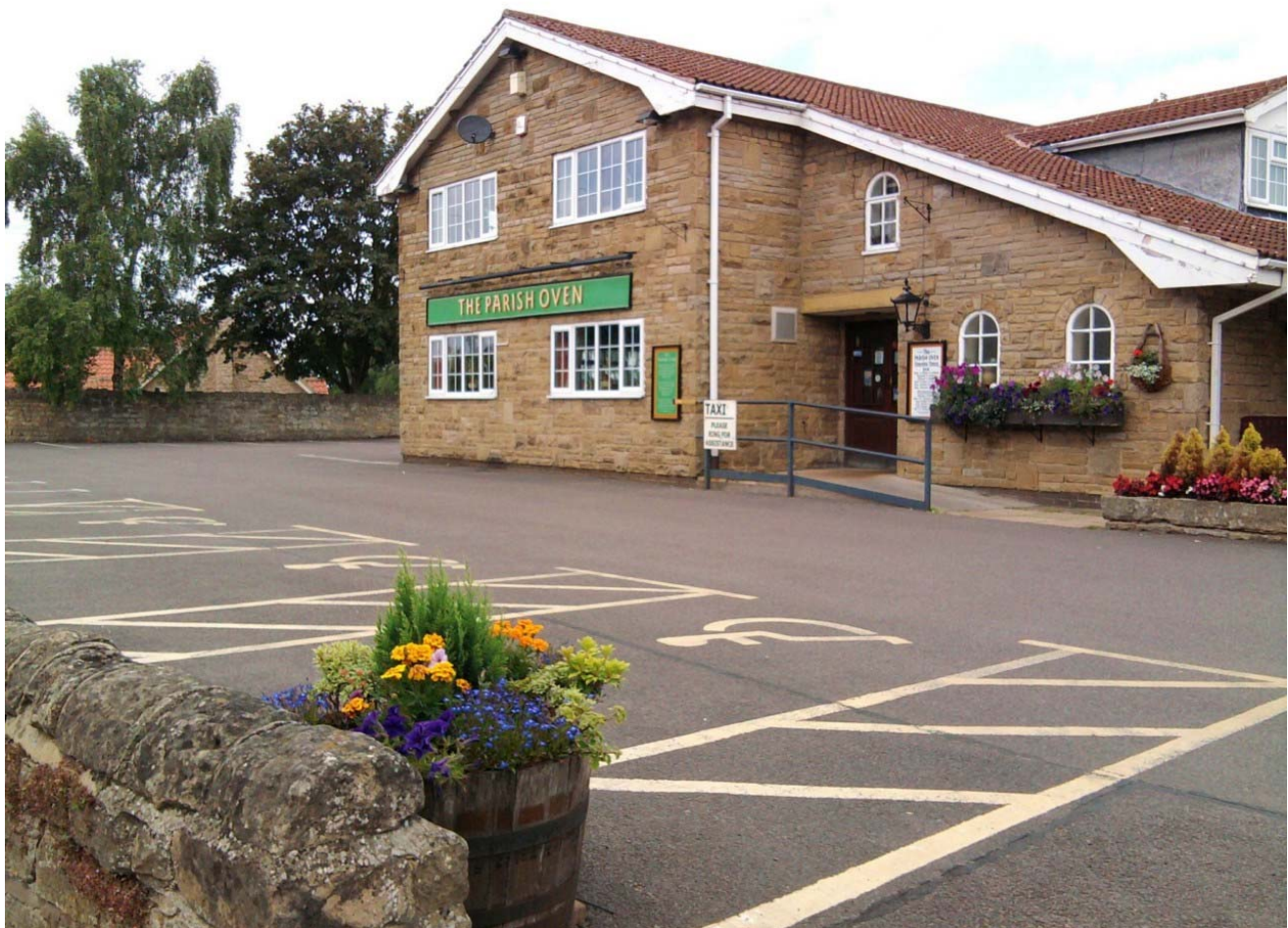
Local Inn 'Parish Oven'
