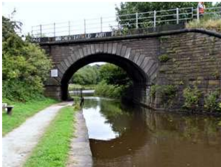
Canal Crushed Stone Towpath
